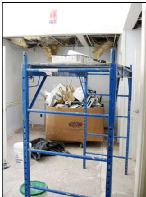
CRHS Health Center second floor waiting room under renovation.
